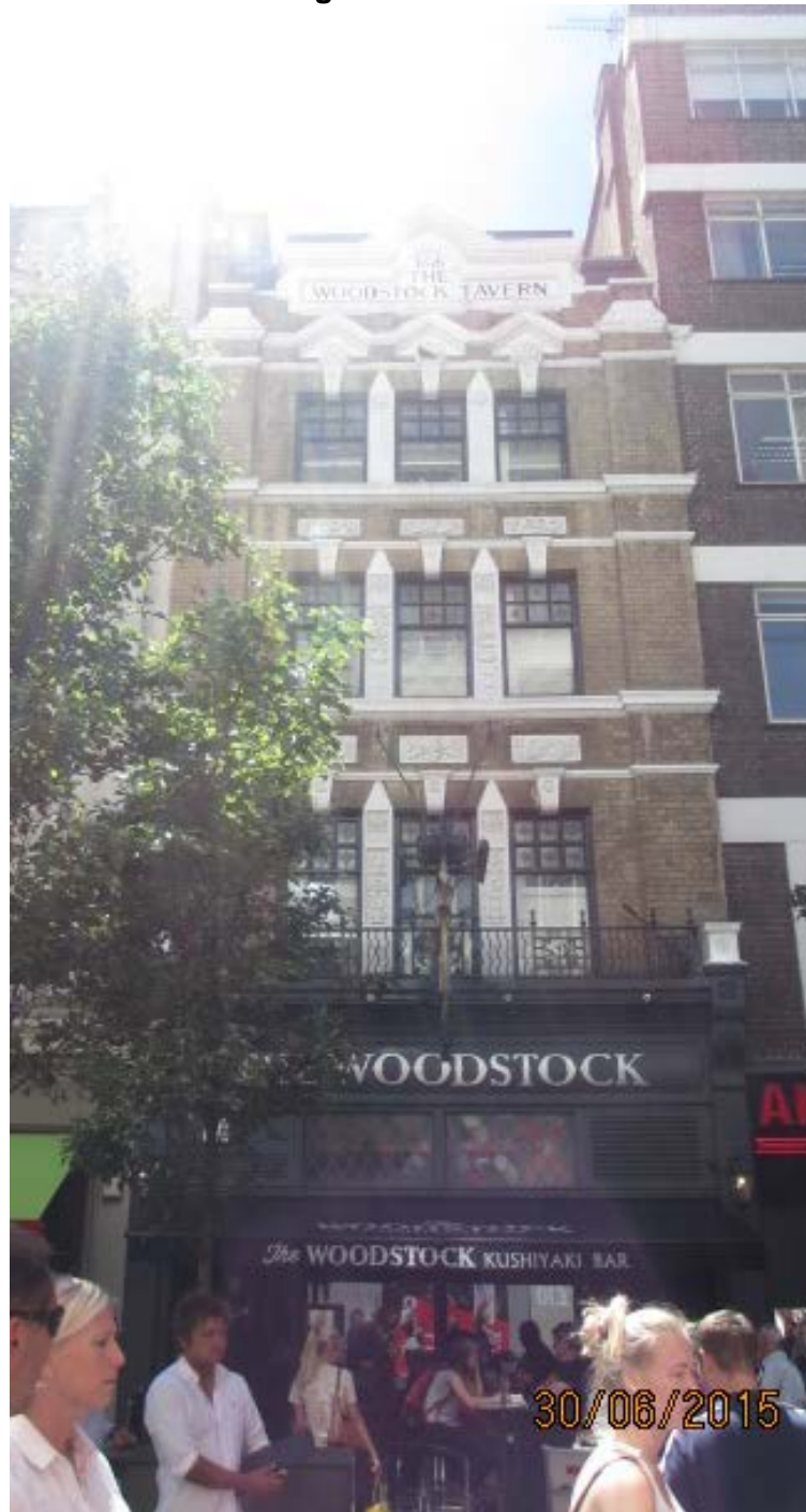
Photograph 1. Front elevation of building
