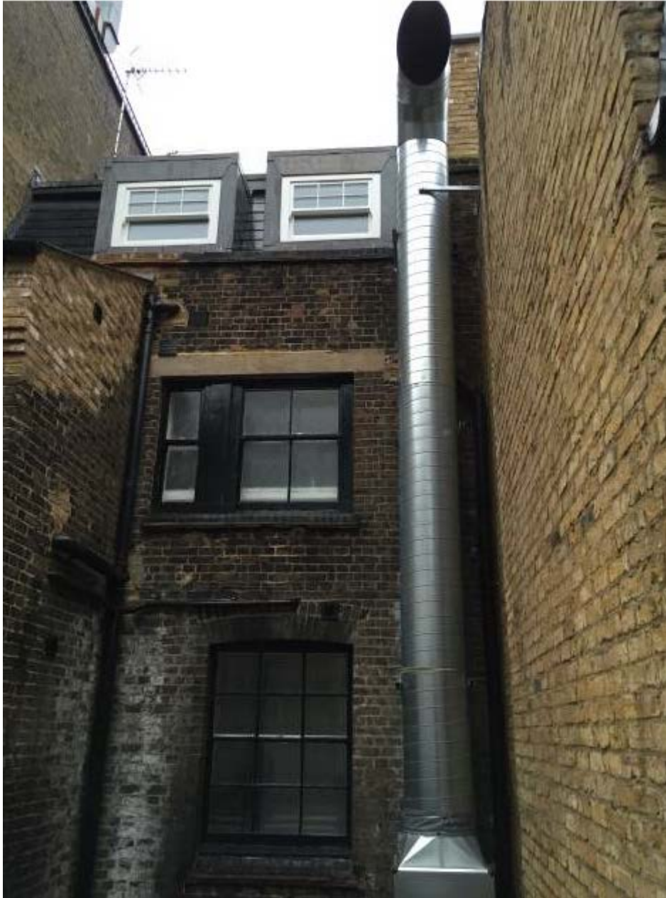
Photograph 2. Duct as installed (between 1 st December 2014 until 18 th July 2016)
